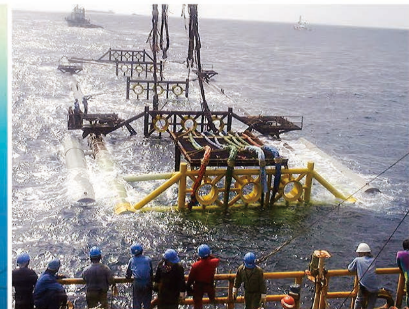
水深90mへの石油生産設備設置工事 Oil production facility installation in 90m water
